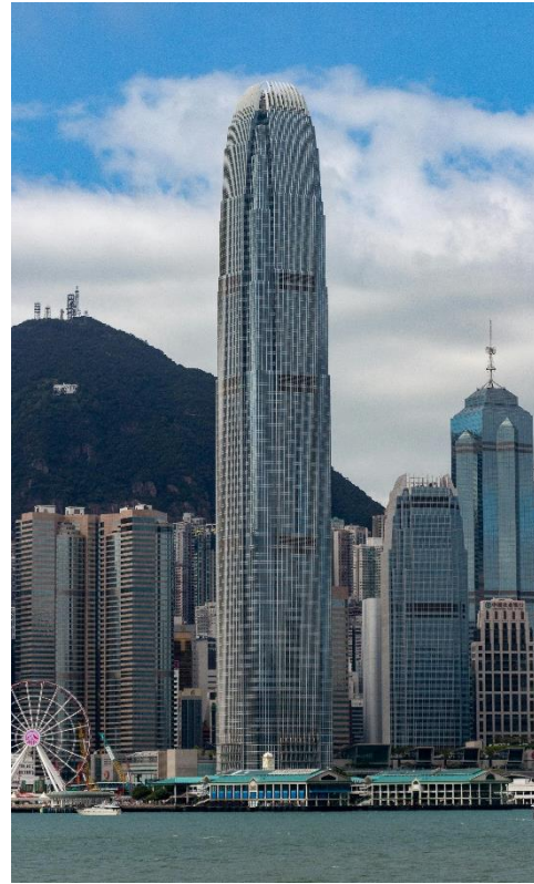
Figura 6: Two International Finance Centre, Hong Kong (2003).
