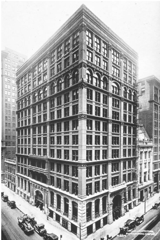
Figura 1: Home Insurance Building, Chicago (1885-1931).
