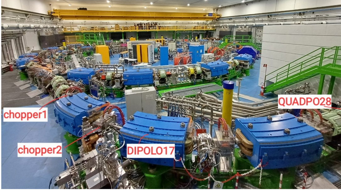
Figure 5.6: Photograph of the initial section of the HEBT in the CNAO synchrotron.
