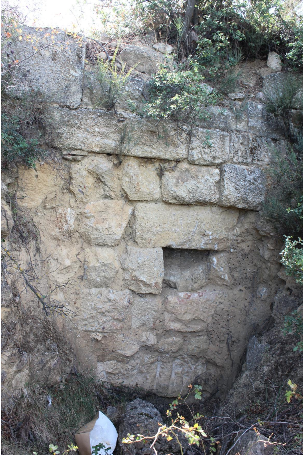
Figure 6, North retaining wall at the acropolis, possibly part of the fortifications, author: EA Kubaska
