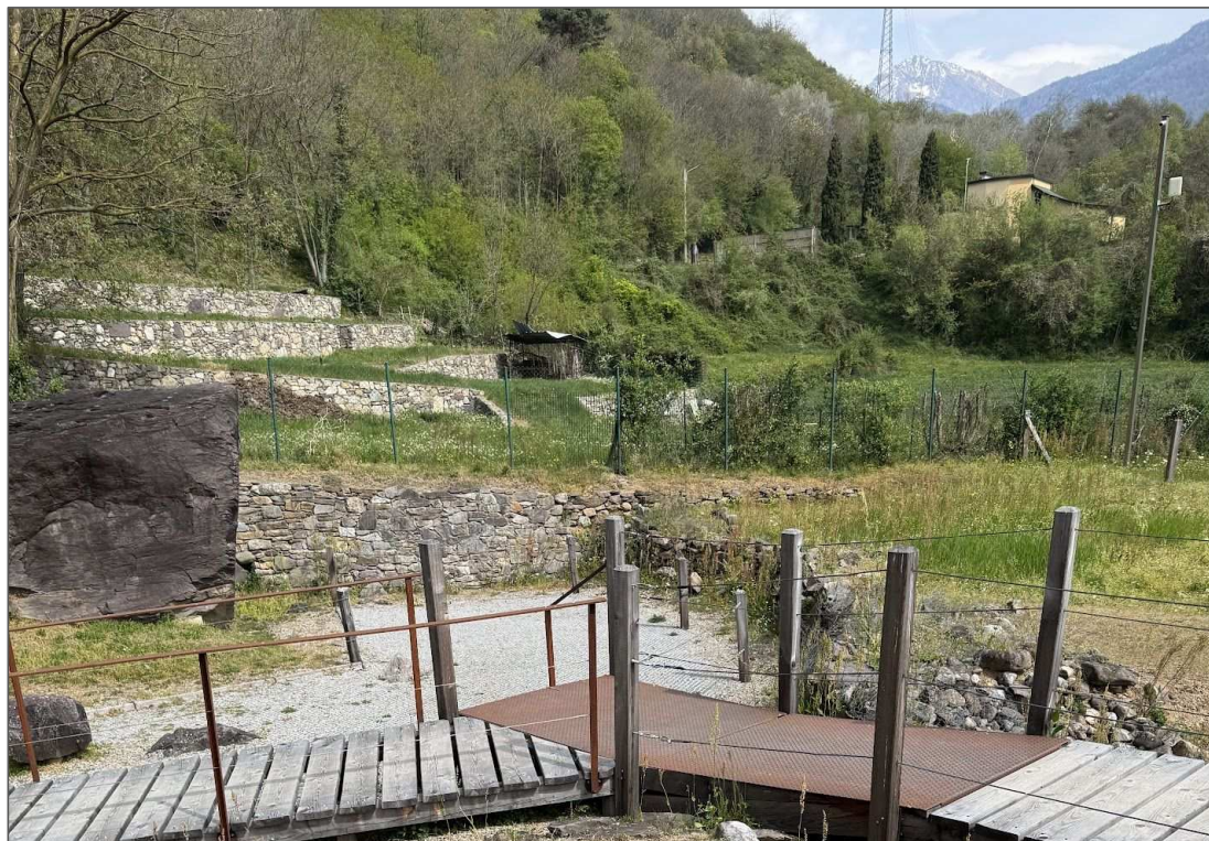
Sanctuary prior to suggested interventions
