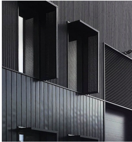
Figure 34: Harwell Zeta – Aluminum shading elements (brise-soleil) reducing solar gain. (Allies and Morrison, n.d.).
