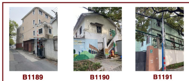
Figure 41: The three buildings show poor envelope conditions and neglect. Their alignment reveals a critical climatic zone where cooling demand is highest.
