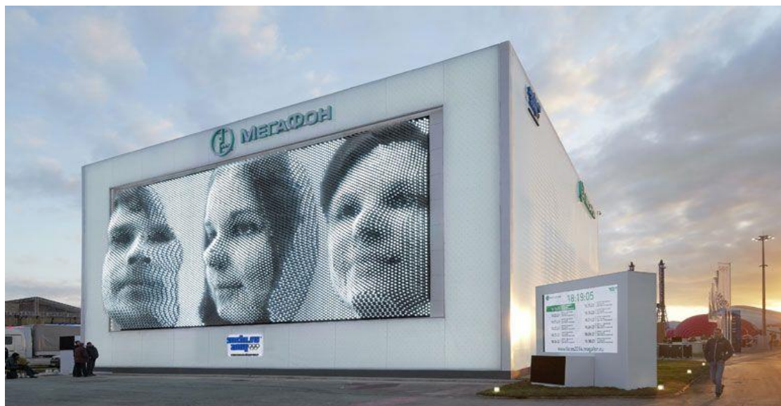
Figure 52 - The MegaFaces pavilion – a 2000 sqm cube created for Russian telecom company Megafon – features a vast kinetic façade that contorts into 3D recreations of visitor's faces, relayed via digital scans made in nearby photo booths.
