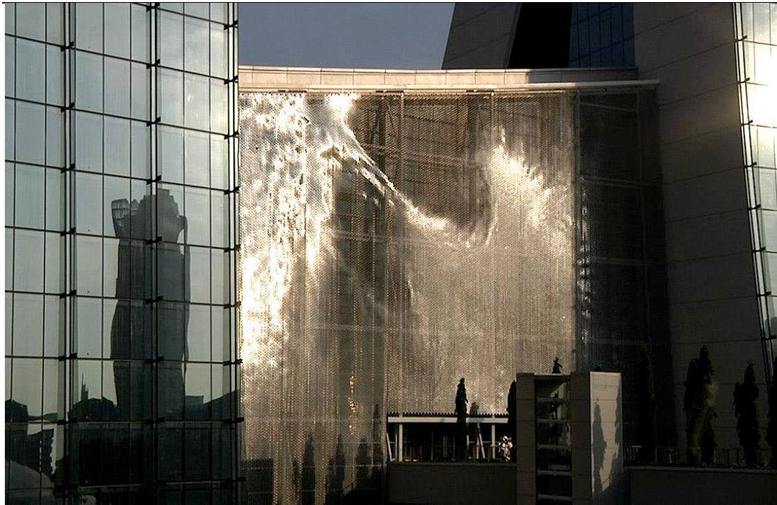
Figure 53 - Wind arbor, a facade of a hotel lobby in Singapore covered with a cable net structure composed of a half a million hinged element
