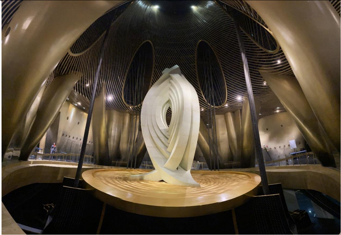
Figure 48 - 1000 metric-ton tuned mass damper that would not only provide an extra guarantee of occupant comfort on the upper floors, but also serve as a tourist attraction
