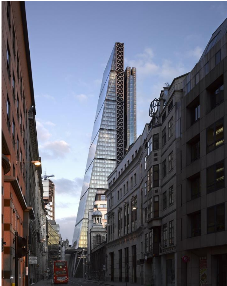
View on the Leadenhall Building, Rogers Strick Harbour + Partners, London, 2014
