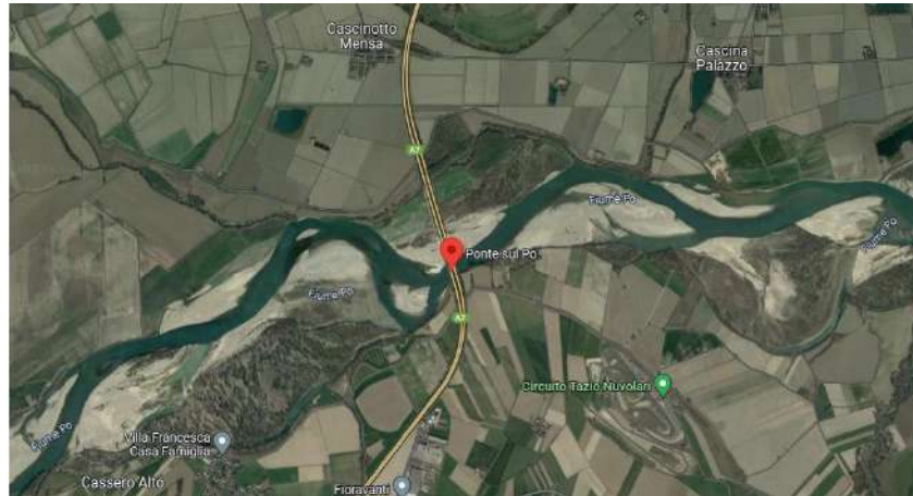
Figure 5.3: Satellite view of the Ponte Po – Careggiata Nord location on the A7 motorway.
