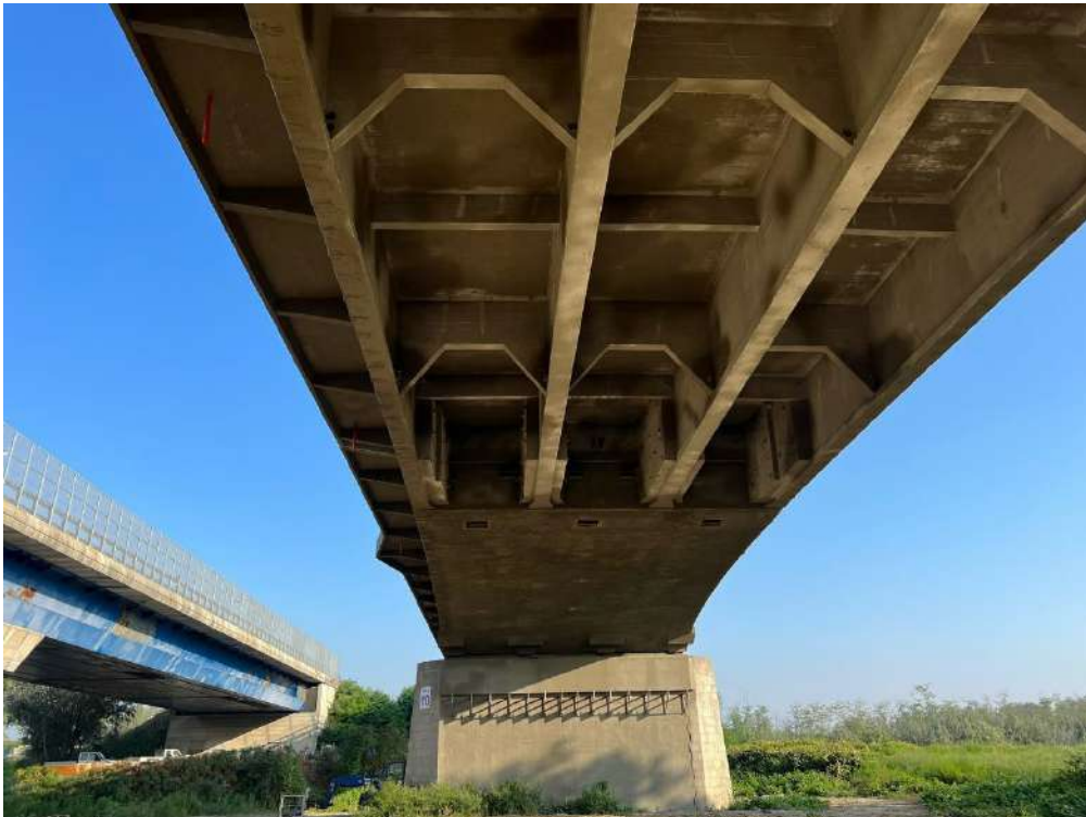
Figure 5.5: Underside structural configuration of the bridge deck showing the girder system.
